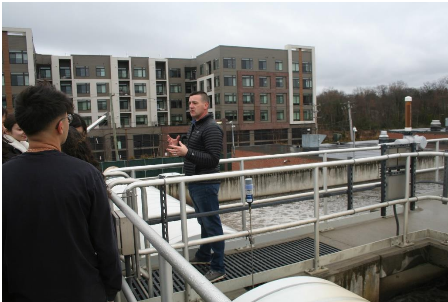
Photo 2 Caption: The GNWPCD's oxidation ditch, where organic compounds in wastewater are consumed, was the third stop made by Superintendent Christopher Murphy along the tour.
