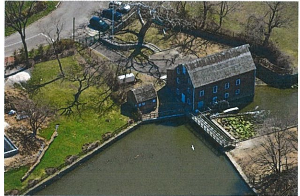
Sewer district replacing damaged pump
