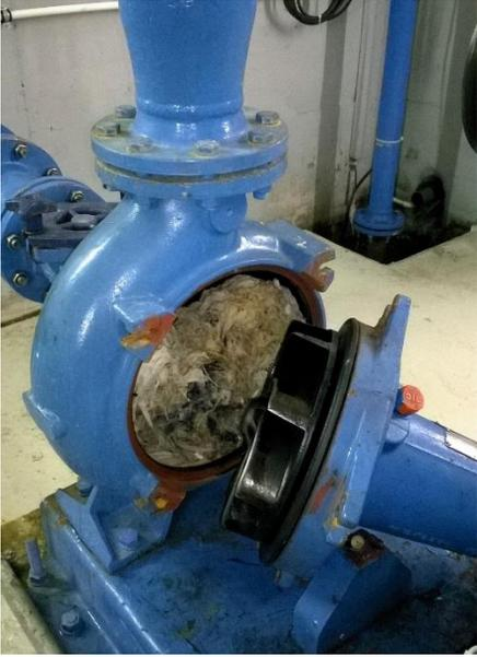
Photo 1: A pump clogged with wet wipes at a wastewater treatment center. (TPO Magazine)
